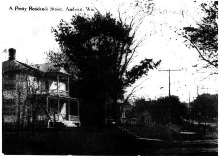
Christ Halvorson's home on Mill Street. Picture taken around 1910.
